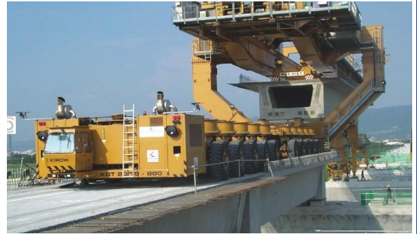
Optical Guided Kirow Multi Mover bridge transporter for elevated highway by Kirow, Germany
